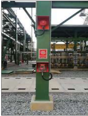
Fire Alarm / Manual call point
